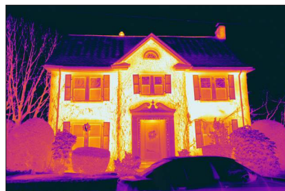
Capturing energy loss from buildings with the drive-by thermal imaging rig.
