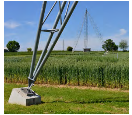
The poles are on massive pillars anchored 3.5 meters deep in the ground.
